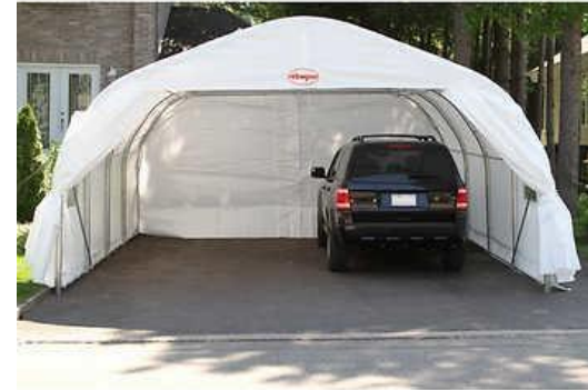
Figure 3.22: Temporary Car Shelter
